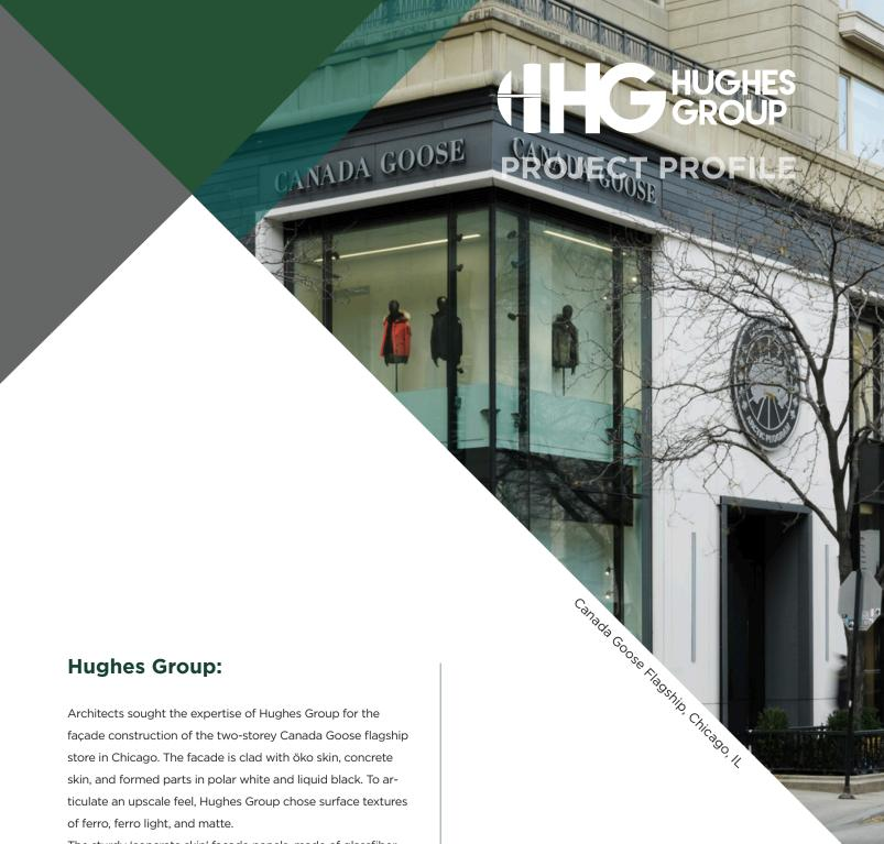
The sturdy 'concrete skin' façade panels, made of glassfiber reinforced concrete, are only 13 mm thin and offered the architect freedom for the design of individual facades. Hughes Group recommend the full Rieder line for its ability to 'wrap' smoothly over buildings, corners, and edges—creating a unique material flow. With öko skin, Hughes Group was able to supply a concrete façade in a slatted design. The various surfaces created a lively interplay of color.
